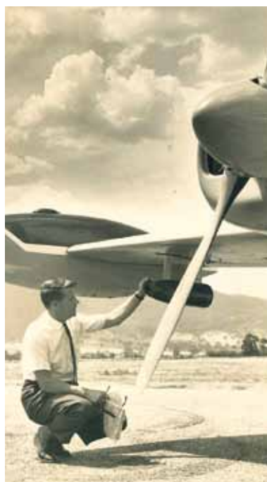
A Cessna aircraft fitted with cloud seeding equipment at Corryong, Victoria in 1966. Photo by Athol Hodgson
